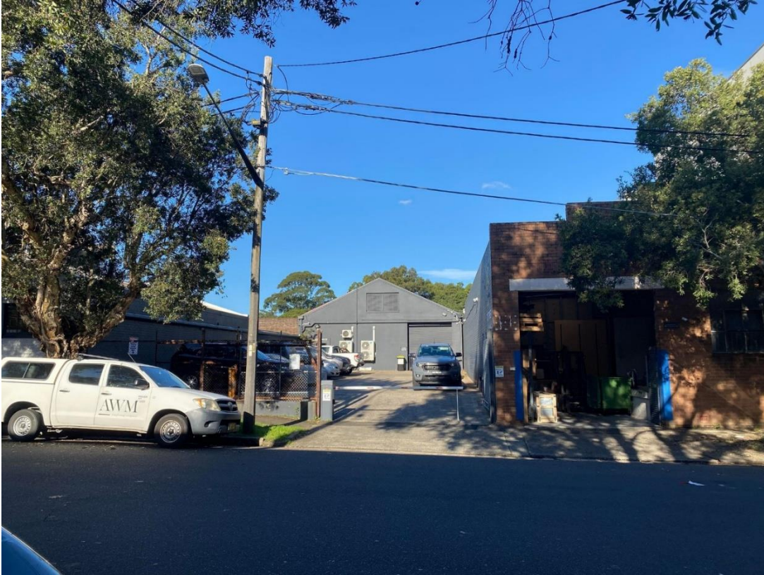
Figure 7: Site viewed from Birmingham Street
