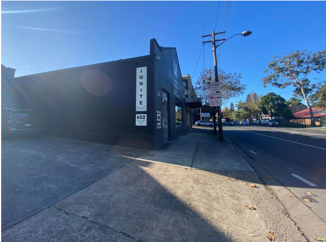
Figure 3: Site viewed from Botany Road looking north
